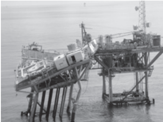
Figure 4.2 A Gulf of Mexico platform after (just) surviving a major hurricane.
