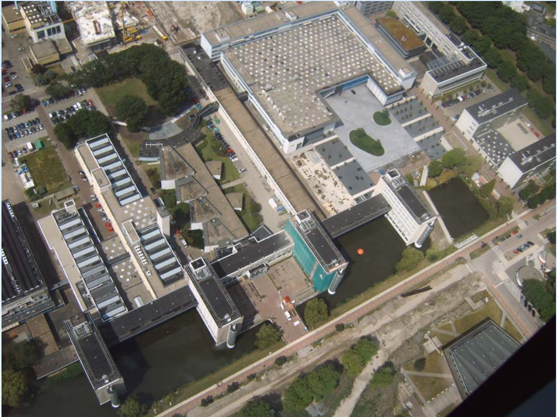
Aerial photograph of Faculty 3mE, Delft University of Technology, Mekelweg 2, Delft
